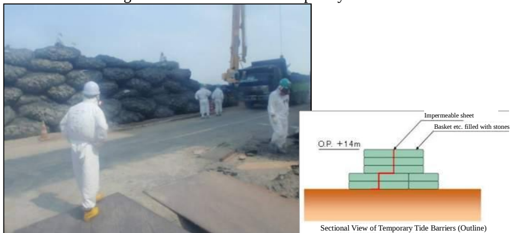
Fig. III-1-8 Installation of Temporary Tide Barriers
